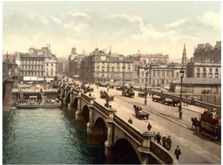
Glasgow Bridge (c.1890s) Wikimedia Commons (CCL)
