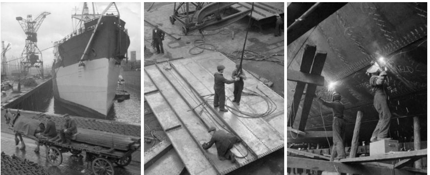
Shipbuilding in Glasgow during the Second World War (1942) Wikimedia Commons (CCL)
